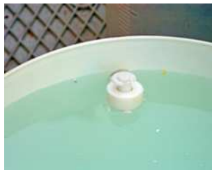
Water level just below the float switch
