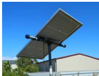
Solar panel mounted on a pole
