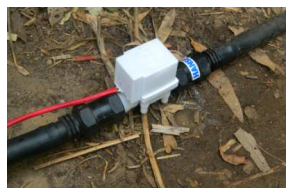
Solenoid valve installed at ground level
