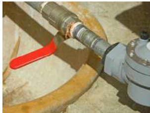
Connect the inlet of the solenoid valve to the water supply
