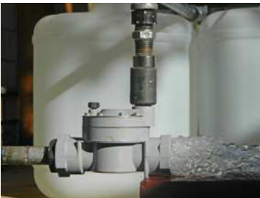
When the magnet is in the low position, the magnet lifts the plunger inside the solenoid and opens the valve
