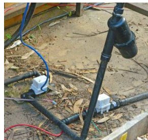
Two solenoids valves, one for each zone
