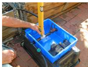
Use a spirit level to ensure that the float shaft is vertical
