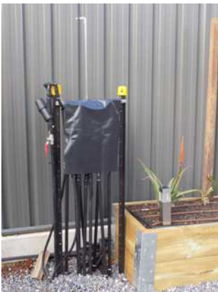
A light-proof cover protects the flow-splitter from algae formation
