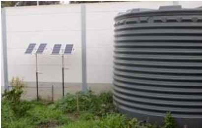
Four 20 watt solar panels provide the power
