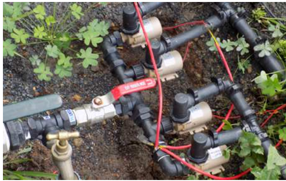
Four 14 watt pumps provide sufficient flow to the flow-splitter 75 metres away and about 4 metres higher
