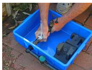
Float shaft must be vertical
