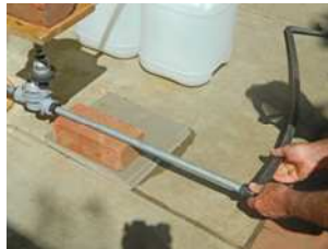
Connect the outlet of the solenoid valve to the irrigation application
