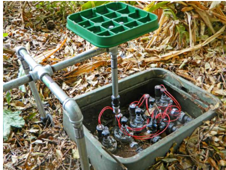
Position the magnet so that it is above the solenoid
