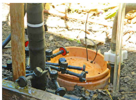
Fraction 1/4 for online dripper (4 closed lower drippers, 4 open lower drippers and
