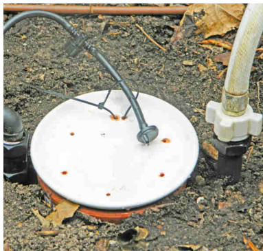
The adjustable control dripper has been replaced by an on-line irrigation dripper.
