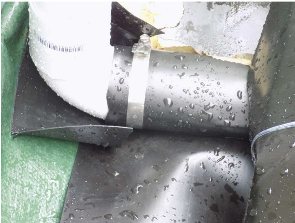
boot connected to rainwater inlet
