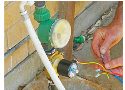
Connect the blue and green wires to the solenoid valve
