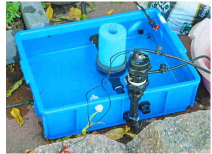
Universal Measured Irrigation Controller used for the fruit tree zone
