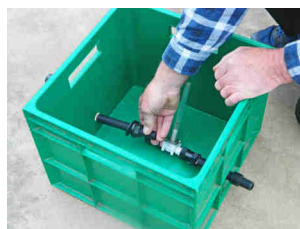
Insert the outlet pipe through the other hole
