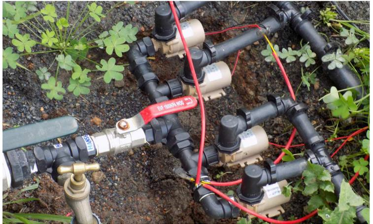
Four 14 watt pumps provide sufficient flow to the flow-splitter 75 metres away and about 4 metres higher
