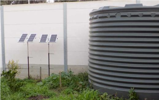
Four 20 watt solar panels provide the power
