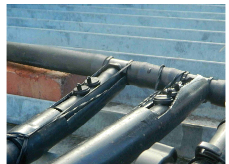
Dripper assemblies for zones 1 & 2 at level 0 on the roof. The drippers are open to the atmosphere.
